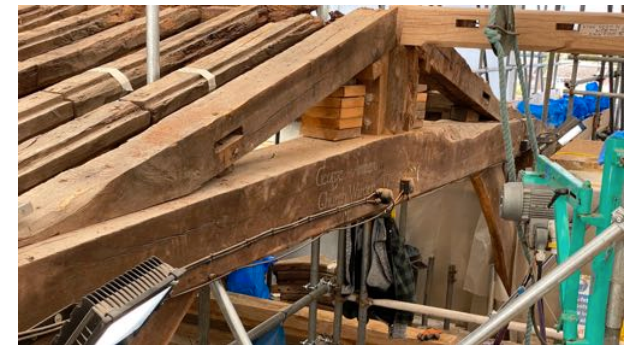
Tie beam, ridge beam & rafter repairs seen during a "Hard Hat Tour"; look closely for an inscribed record of past works in 1791
